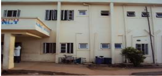
Fig 3: Littered Hospital environment
