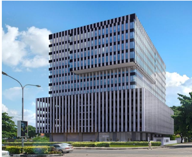
Figure 2 – The Heritage Place in Ikoyi Lagos (Actis Group, 2016)
