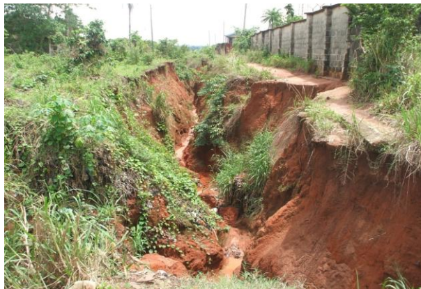
PLATE 1: Works layout road threatened by gully (source: authors field work 2016) Gully Erosion Development Process
